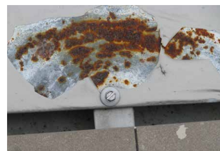
When the paint is removed corrosion down to base steel is clearly visible.
