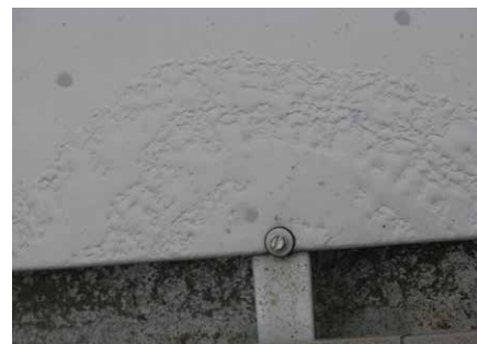
Paint bubbling radiating out from stainless steel fastener on roof 300ft from ocean.
