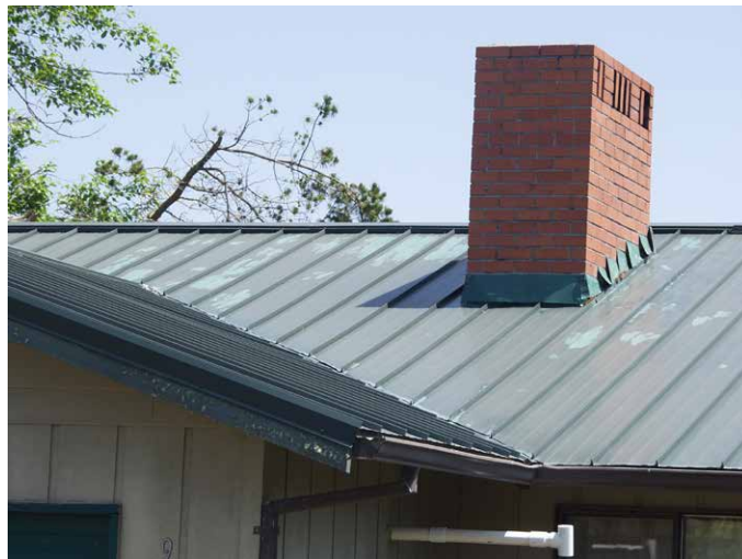
Excessive use of touch-up paint that has faded faster than factory applied coating.
