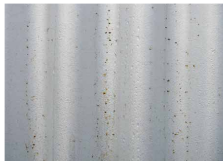
Moderate swarf staining on ZINCALUME Plus.
