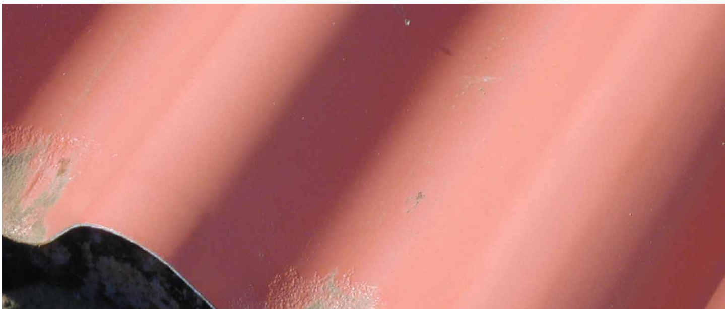
Silt accumulation on a panel without a drip edge. Blistering of the paint is an early sign of corrosion.
