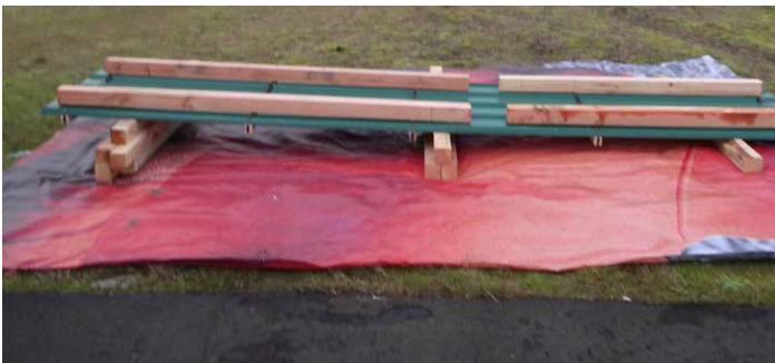
Scrap material used to keep tarp from resting directly on bundle.
