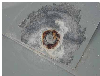
Over driven fastener resulting in premature corrosion of the ZINCALUME panel.
