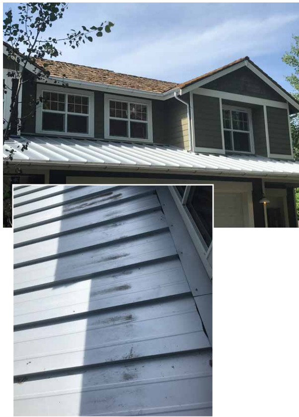
Copper treated shingles above bare ZINCALUME roof panels, the water runoff resulted in black oxidation.
