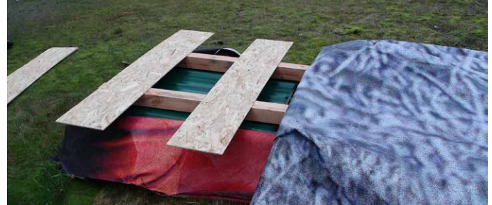
Tarp rolled over stack with a minimum of 12" overlap on all sides.
