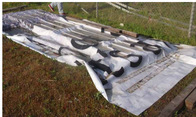
Improper Storage - By snugly fitting a tarp directly on the ground.
