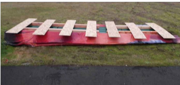
Tarp edges rolled up and hole cut in lowest area of tarp to allow water to escape.
