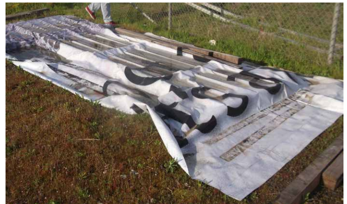
Improper Storage - By snugly fitting a tarp directly on the ground.
