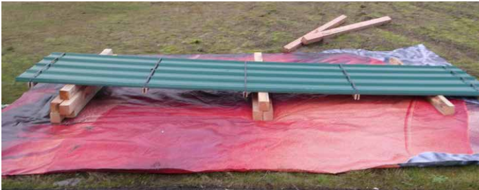
Bundle placed in a sloping position to gravitate moisture out.
